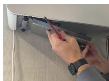
**3:** Install the drain hose with heating element. Insert the plug and reinstall the metal cover as shown:
